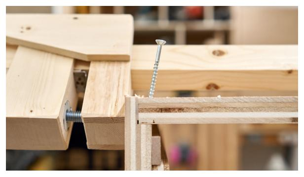
Be careful not to make the angle too sharp, or the screw will go through the side of the cabinet. It might be helpful to draw a line on the front edge of the side panel to guide the bit while drilling the pilot hole.
